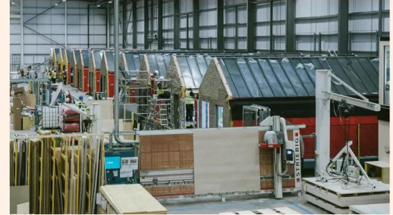
TopHat puts together rooms, units or entire houses on a factory line, which is more automated so the developer can scale at pace © TopHat
