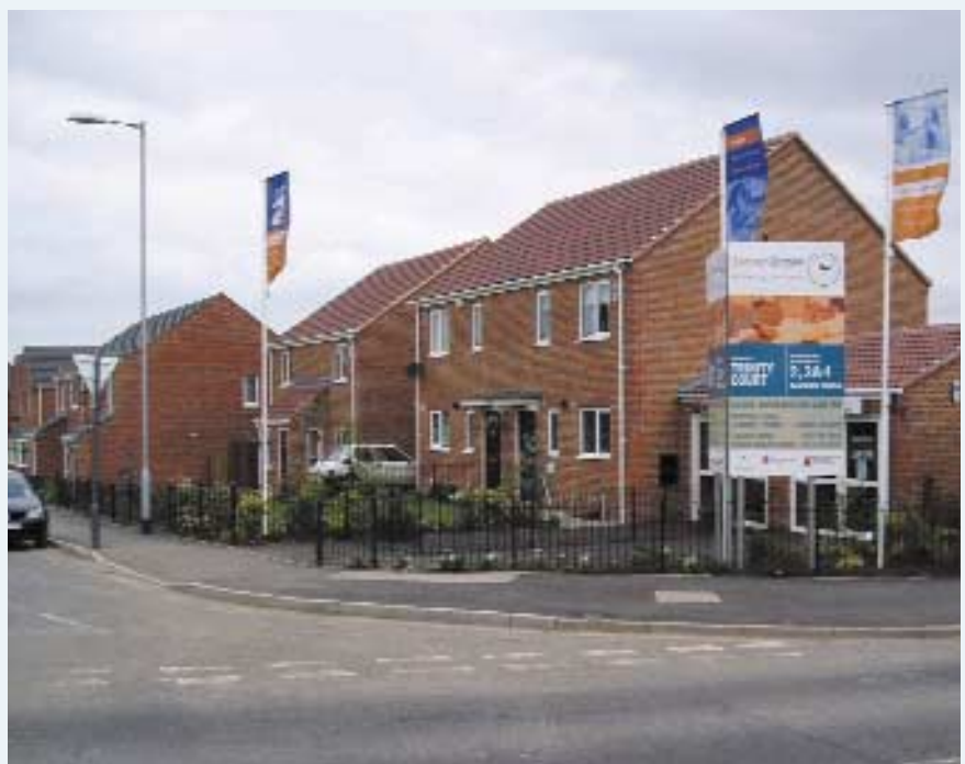
Working in partnership with housing providers
