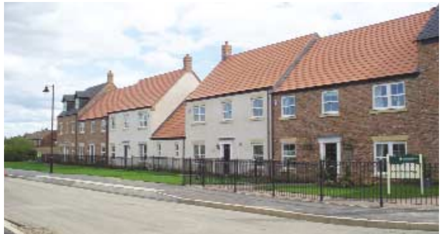
Family housing at Newcastle Great Park
